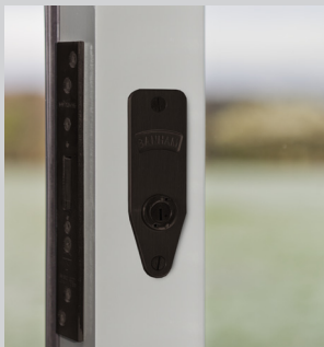
BANHAM LOCK WITH ESCUTCHEON PLATE
