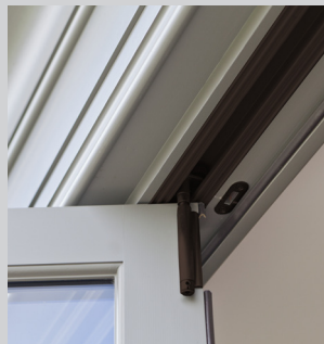
TOP TRACK AND CARRIER HINGE
